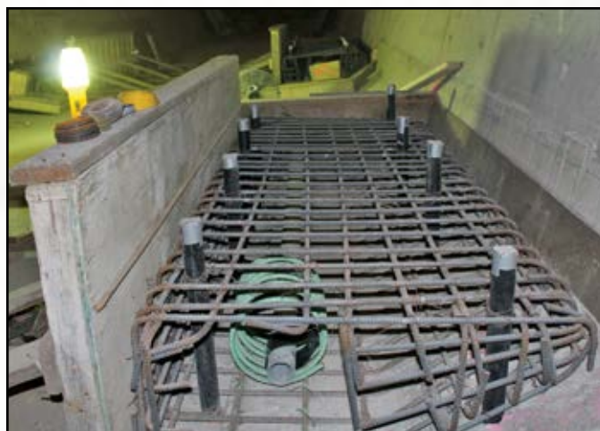
Project: Muskegon River Bridge Contractor: Freyssinet USA Location: Big Rapids, MI
