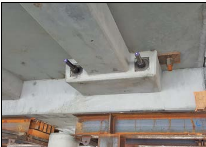
Project: SR 520 Evergreen Point Floating Bridge General Contractor: Kiewit/General/Manson, JV Post-Tensioning Supplier: Schwager Davis, Inc. Location: Seattle, WA
