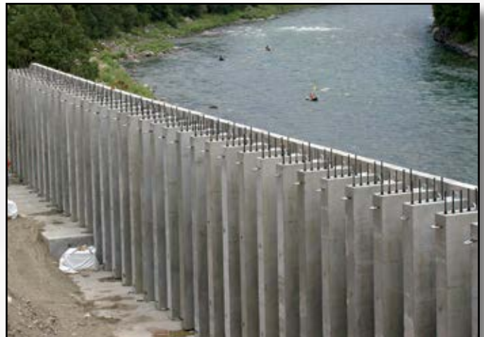
Project: Precast Post-Tensioned Panel Wall Contractor: Morgan & Oswood Location: Hoback Junction, WY
