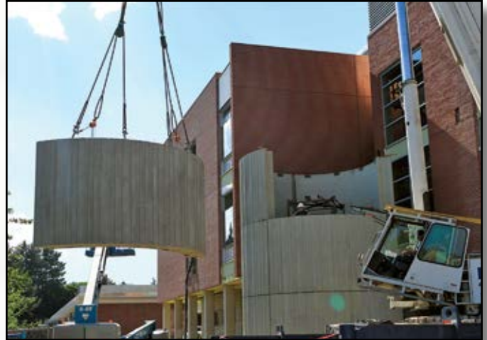
Project: Astronomical Observatory Tower Contractor: Narum Concrete Construction Location: Central Washington University, Ellensburg, WA
