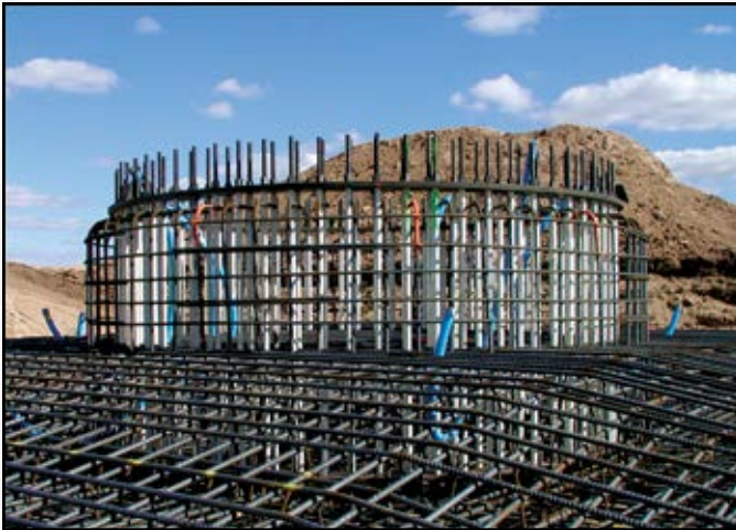
Project: Peetz Colorado Contractor: Blattner Energy Inc. Location: Peetz, CO
