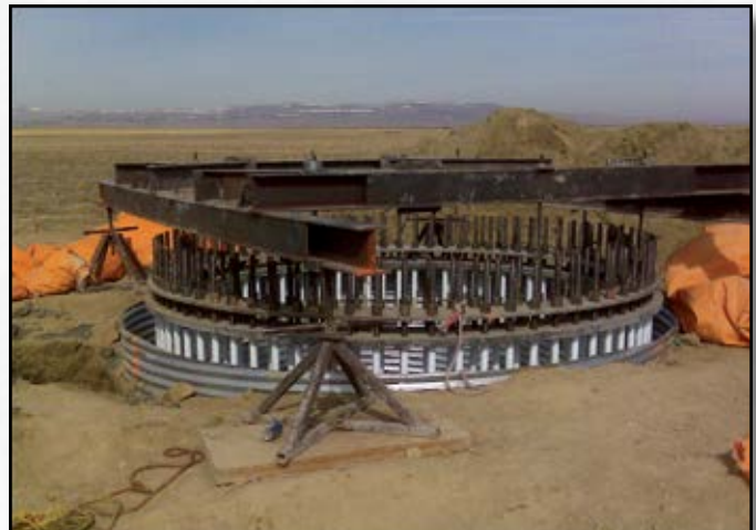
Project: Blue Trail Wind Farm Contractor: TransAlta Location: Ft. Macloed, AB
