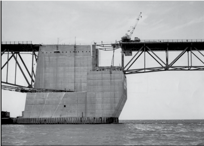
Project: Mackinaw Bridge Contractor: Merritt-Chapman & Scott Corp. Location: Mackinaw, MI
