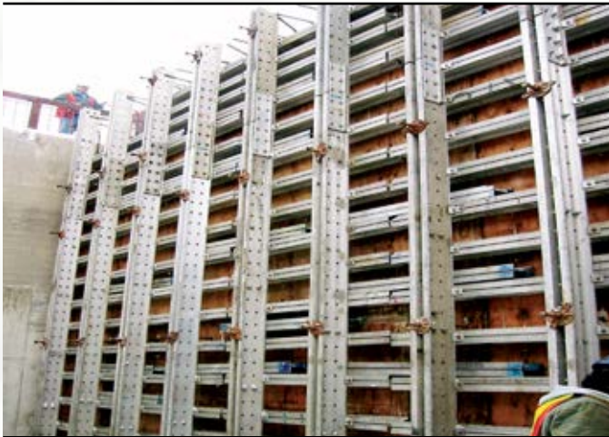
Project: Windsor Pumping Station Contractor: Oscar Construction Inc. Location: Windsor, Ontario
