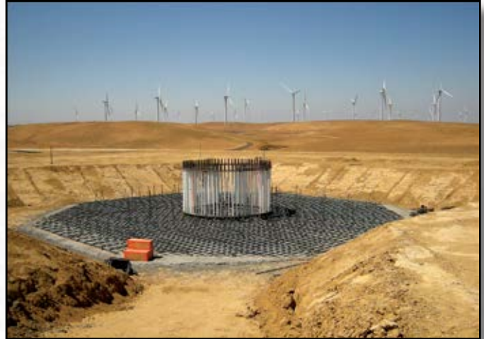
Project: Shilo II Wind Farm Contractor: M.A. Mortenson Co. Location: Rio Vista, CA Photo: enXco & Mortenson Co.
