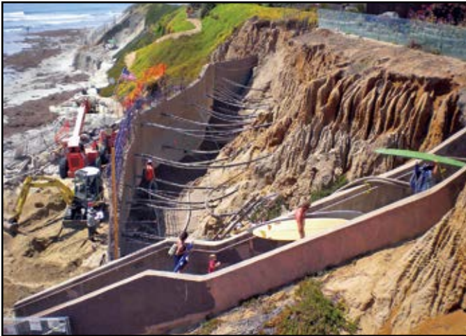
Project: Igor's Seawall Contractor: R&R Drilling Location: Carlsbad, CA
