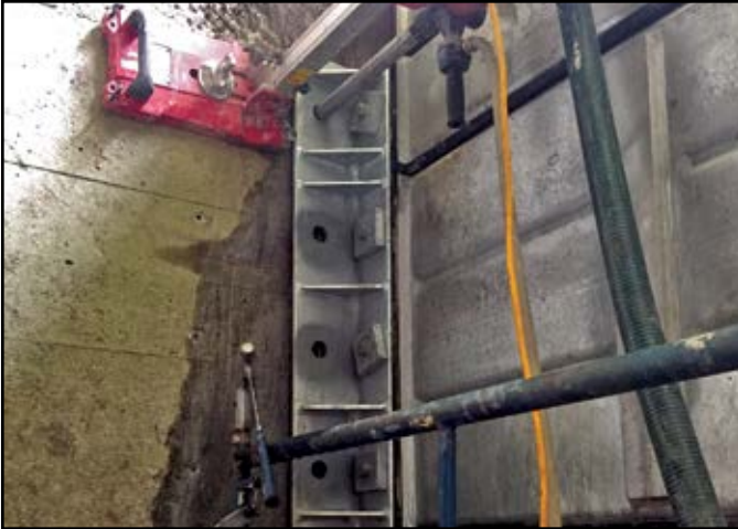
Project: Bridge River 1 Stoplog Contractor: BC Hydro Location: Shalath, BC
