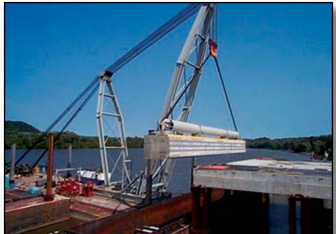
Project: London Lock & Dam Rehabilitation Contractor: OCCl Inc. Location: London, WV
