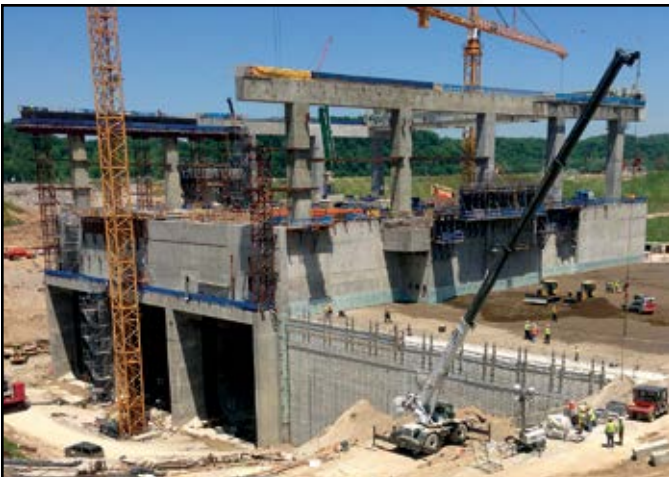
Project: Cannelton Hydro Contractor: Walsh Construction Location: Hawesville, KY
