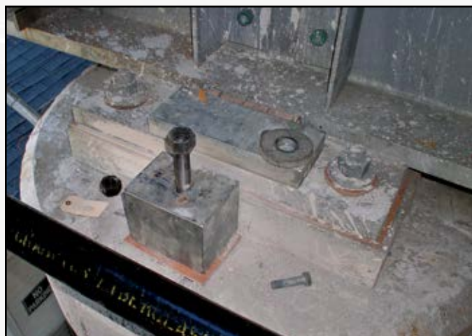
Project: Chicago Elevated Train Contractor: Kiewit Location: Chicago, IL
