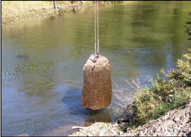
Project: CSX Concrete Removal Contractor: Fenton Rigging Location: Benton Harbor, MI
