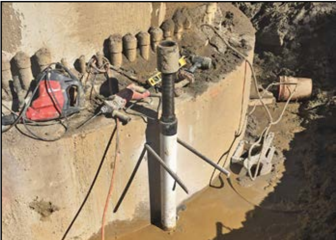
Project: Foundation Upgrade Contractor: JBS Energy Solutions Location: Mountaineer, WV
