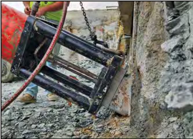
Project: University of Cincinnati Indoor Practice Facility Engineer: Scherzinger Drilling Location: Cincinnati, OH
