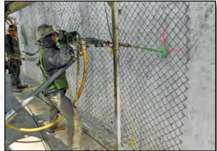
Project: Thornton Reservoir Contractor: Walsh Construction Location: Thornton, IL
