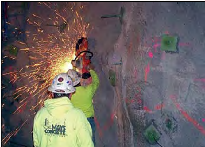
Project: 1-70 Hanging Lake Tunnel Cross Passage Contractor: Mays Constuction Specialties Inc. Location: Glenwood Canyon, CO
