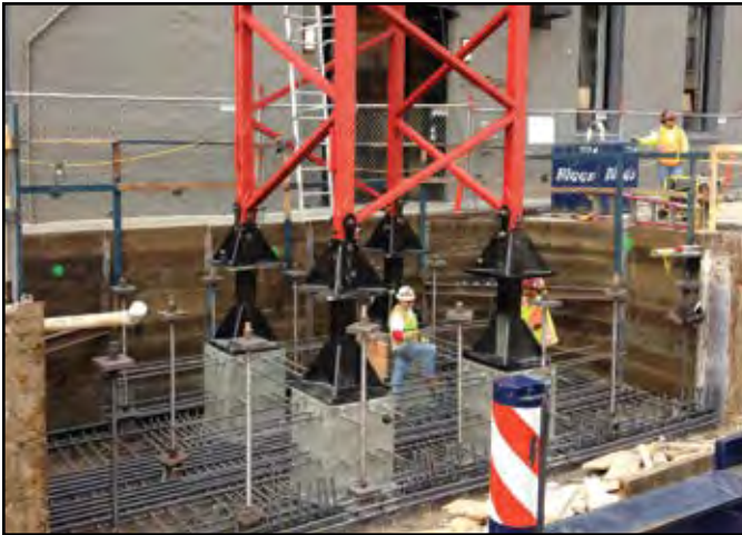
Project: 535 Mission Contractor: Malcolm Drilling Location: San Francisco, CA
