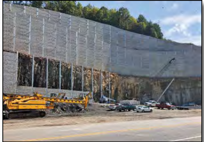
Project: Morgan Roane Hwy Contractor: GeoStabilization International Location: Tennessee
