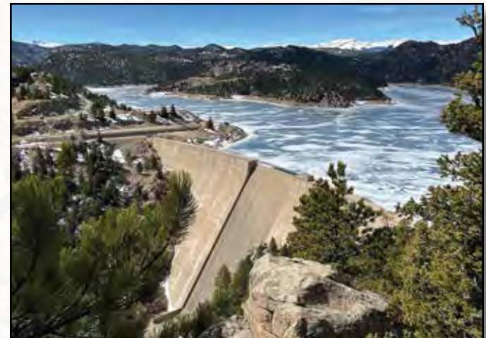
Project: Gross Reservoir Dam Contractor: Kiewit Corp. Location: Boulder County, CO
