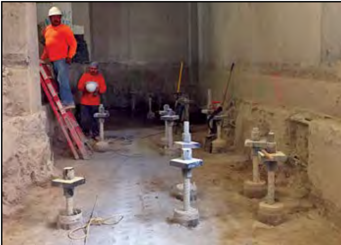
Project: UCSD Contractor: Condon-Johnson & Associates Location: San Diego, CA
