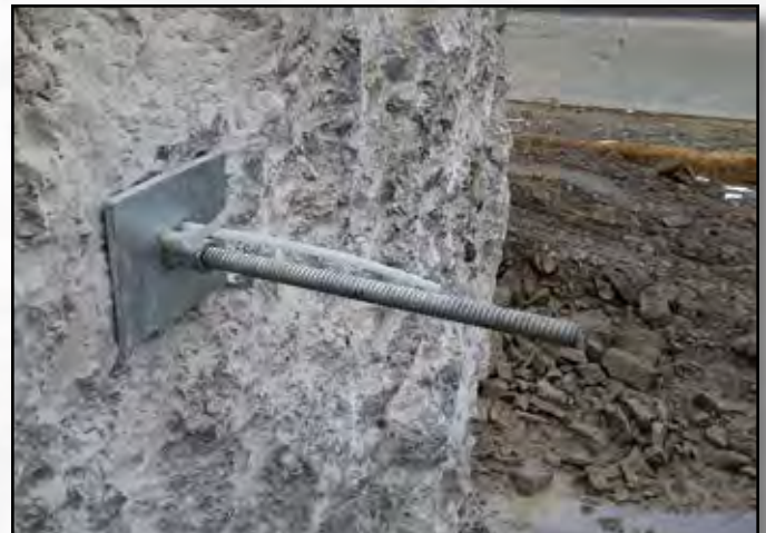
Project Name – St. Lawrence Seaway Lock 5 Contractor – Rankin Construction Inc Location – St. Catharines, ON
