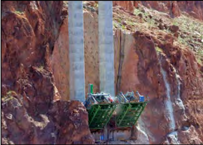
Project: Hoover Dam Bypass Bridge Contractor: Obayashi/PSM Rock Anchors Subcontractor: Roy E. Ladd & Assoc. Location: Boulder City, NV
