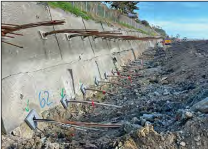
Project: OCTA Landslide Repair Contractor: Condon Johnson Location: San Clemente, CA
