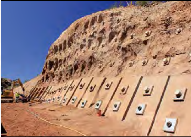
Project Name: Boulder Highway Contractor: GSI Location: Boulder City, NV
