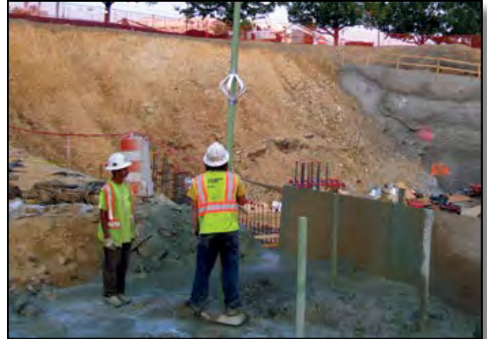
Project: NASCAR Hall of Fame Contractor: Hayward Baker Location: Charlotte, NC
