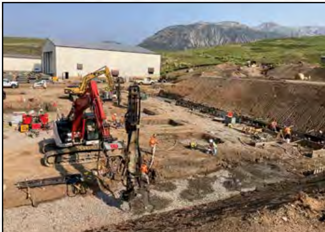
Project: Telluride Airport Contractor: Mays Construction Specialties Location: Telluride, CO
