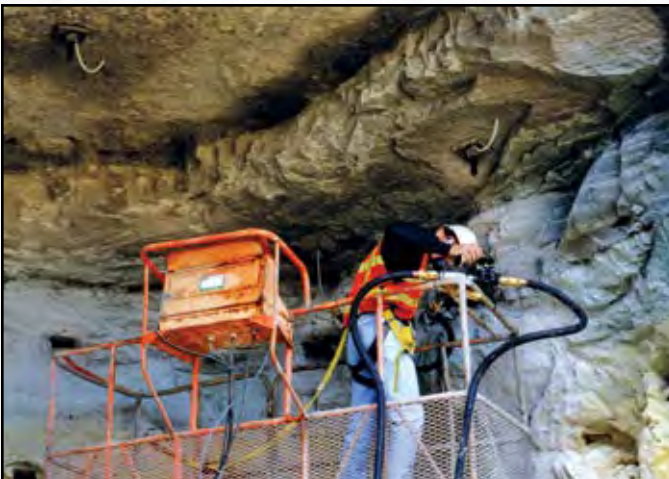
Project Name – University of Minnesota Archive Storage Contractor – CS McCrossan Location – Minneapolis, MN
