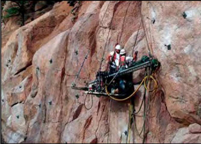
Project: Slope Stabilization Contractor: Yenter Companies Location: Cheeseman Reservoir, CO
