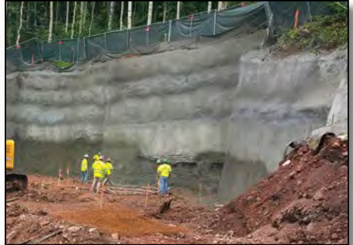
Project: Private Residence Contractor: GeoStabilization International Location: Colorado
