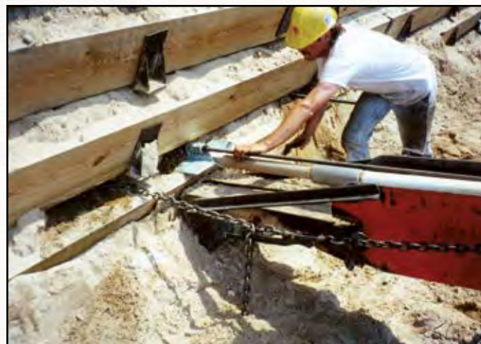
Project: Van Andel Hospital Contractor: King Co. Location: Grand Rapids, MI
