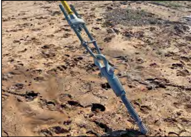
Project: SunZia Transmission Contractor: Crux Subsurface. Location: Arizona & New Mexico
