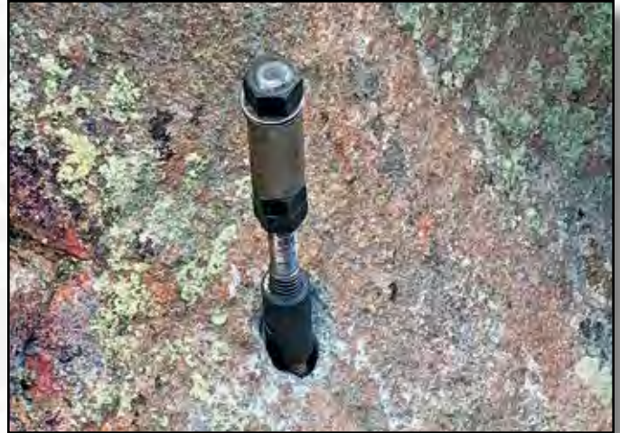
Project: Mill Hnd Transmission Line Contractor: Xcel Energy Location: Silverthorne, CO
