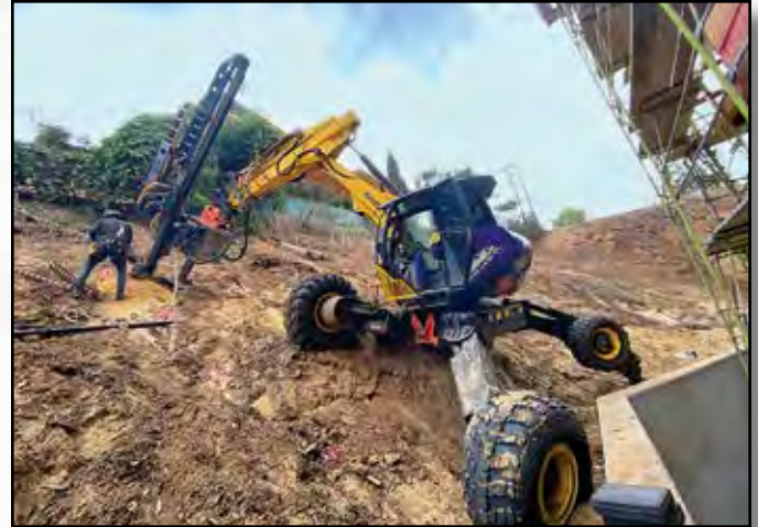
Project: Sepulveda Blvd Contractor: Access Limited Location: Los Angeles, CA
