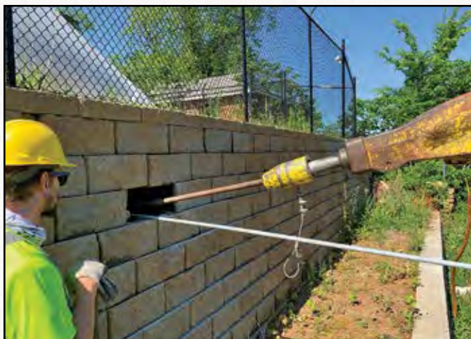
Project: Atlanta Air Dome Location: Atlanta, GA
