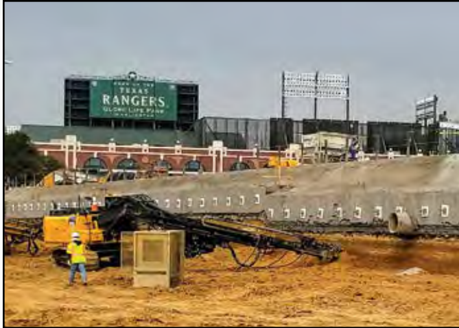
Project: Globe Life Park Contractor: Keller Location: Arlington, TX
