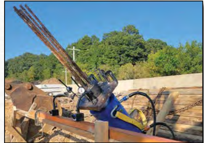
Project: Spavinaw Creek Causeway Contractor: Foundation Specialties Location: Lake Eucha, OK
