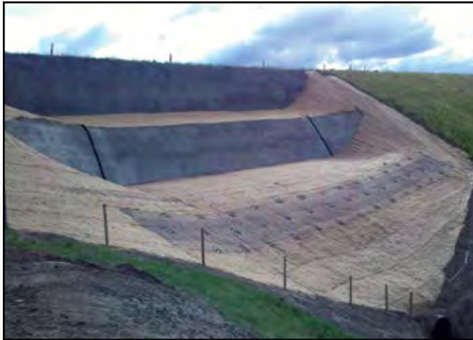
Project: Landslide Repair Contractor: GeoStabilization Incorporated Location: Geyser, MO
