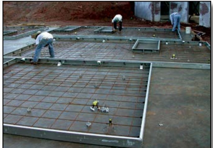
Project: Wakulla County Prison Contractor: Fast Form International Location: Crawfordville, FL
