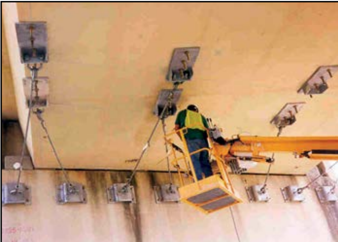
Project: Seismic Retrofit TDOT Contractor: St. Louis Bridge Location: Tennessee
