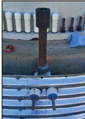
Project: Foundation Upgrade Contractor: JBS Energy Solutions Location: Mountaineer, WV
