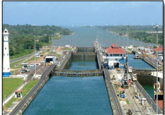
Project: Panama Canal Rehab Contractor: Panama Commission Location: Panama Canal, Panama
