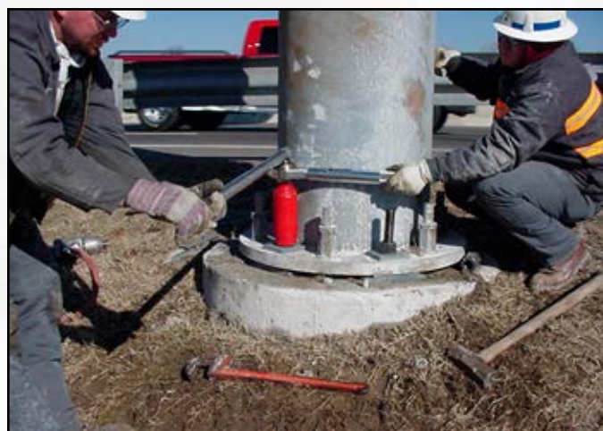
Project: Tennessee DOT Cantilever Sign Retrofit Contractor: Thompson & Thompson Location: Throughout Tennessee
