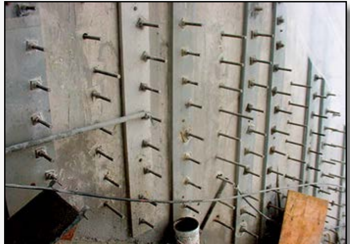
Project: Pineview Dam Contractor: Cal Wadsworth Location: Ogden River, UT
