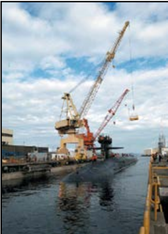
Project: Navy Ship Yard Fender Repair Location: Bangor, WA
