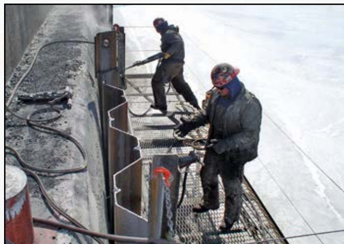
Project: Marine Terminal Contractor: Toledo Caisson Location: Toledo, OH
