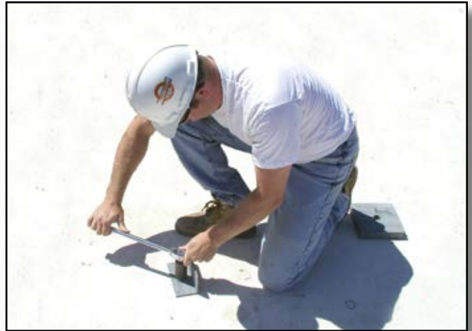
Project: S-7 Installation Testing Location: Grand Rapids, MI
