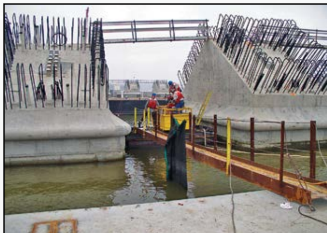
Project: Woodrow Wilson Bridge Contractor: American Bridge Location: Washington DC
