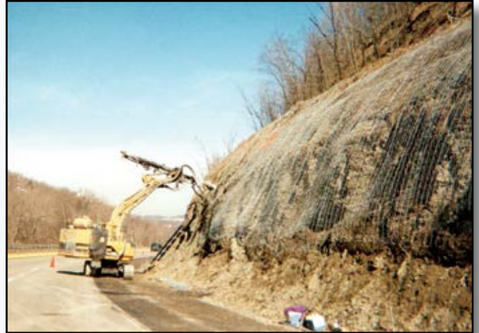
Project: 51 West End Bypass Contractor: Baker Heavy Highway Location: Pittsburgh, PA
