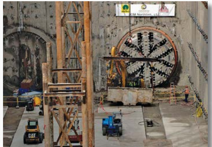
Project: Seattle Northgate Link Extension Contractor: DBM Location: Seattle, WA
