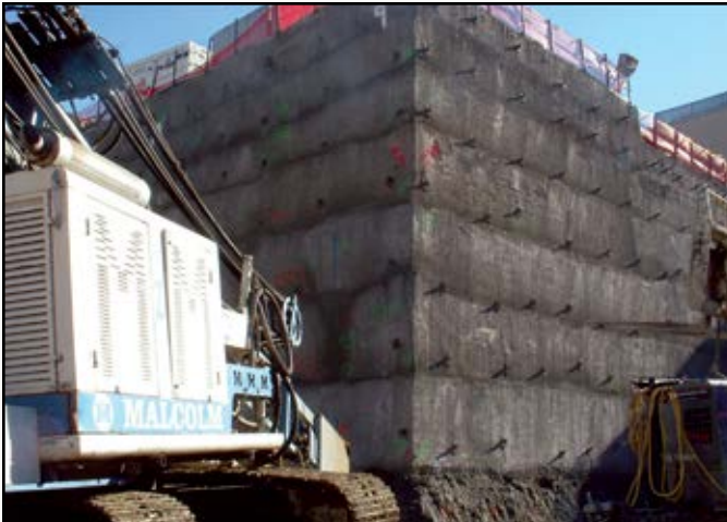
Project: Bravern Towers Contractor: Malcolm Drilling Location: Seattle, WA
