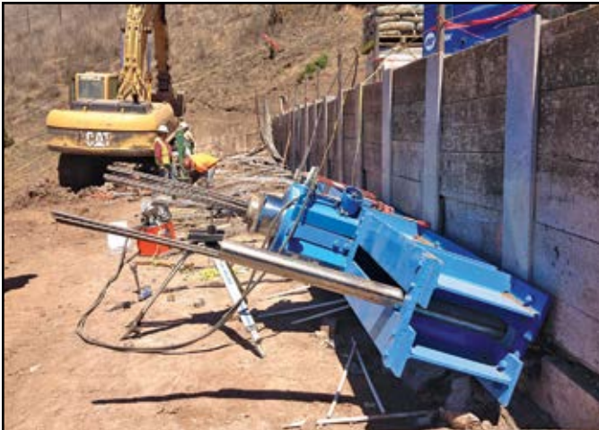
Project: Wilson Landslide Project Engineer: Malcolm Drilling Location: Berkeley, CA
