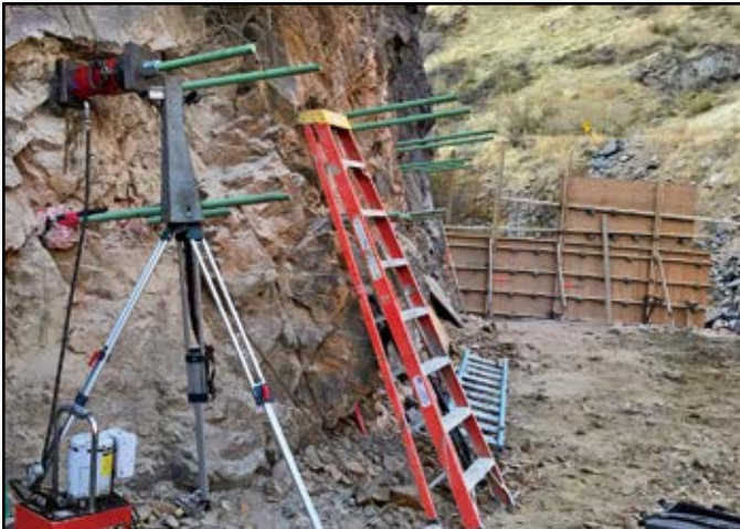
Project: Peaks to Plains Trail Contractor: Midwest Rockfall Location: Golden, CO
