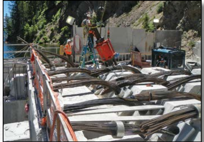
Project: Hebgen Dam Contractor: Jensen Drilling Location: Hebgen, MT
