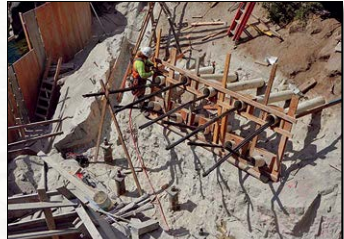
Project: Manning Crevice Bridge Contractor: Inland Foundation Specialties Location: Riggins, ID
