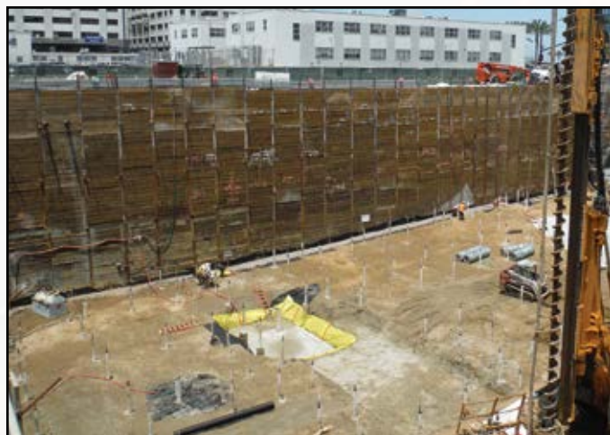
Project: Broadway and Pacific Contractor: Condon-Johnson & Associates Location: San Diego, CA
