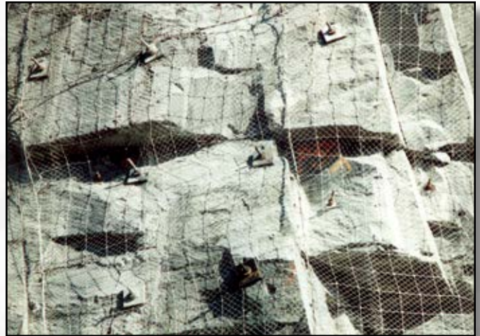
Project: Nantahala Dam Contractor: Boyles Brothers Location: Ashville, NC
