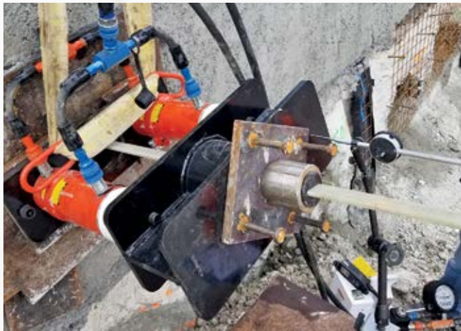
Project: Texas State Capital Bldg Contractor: Oscar Orduno, Inc. Location: Austin, TX
