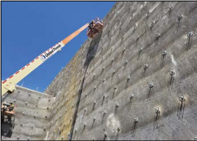
Project: Globe Life Field Contractor: Keller Location: Arlington, TX
