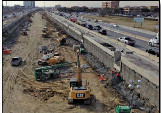
Project: Interstate 635 Contractor: Craig Olden Location: Dallas, TX
