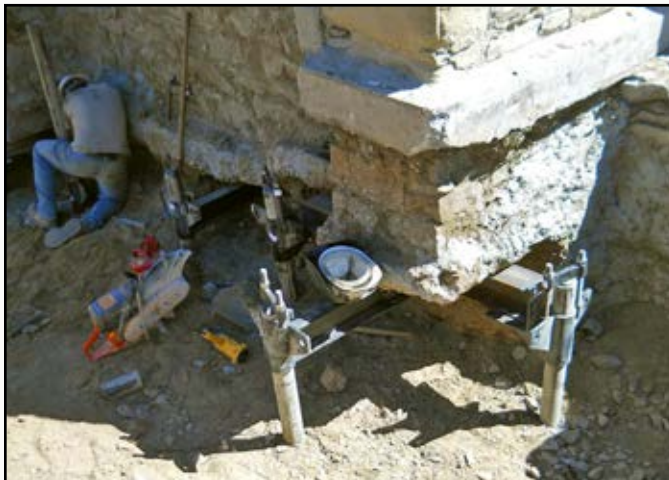
Project: Wyoming State Capitol Contractor: Straight Line Construction Location: Cheyenne, WY
