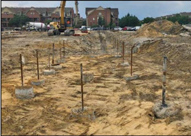
Project: Mix Use Building Contractor: Hardman Construction Location: Royal Oak, MI
