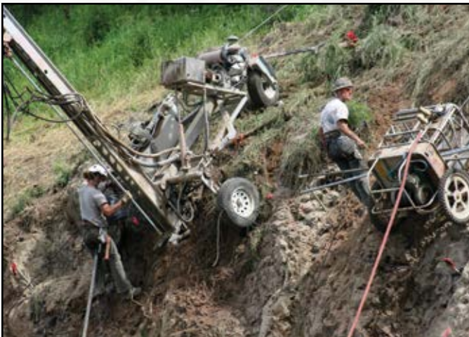
Project: Hana Highway Contractor: Prometheus Construction Location: Maui, HI
