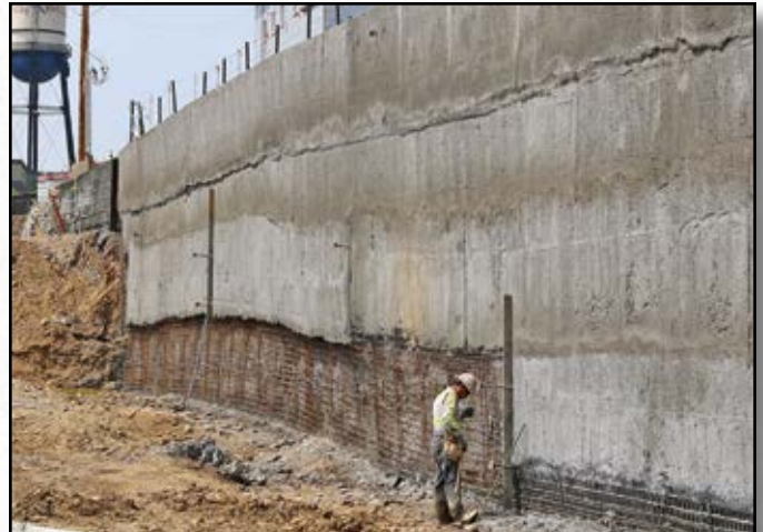
Project: Arvada Parking Garage Contractor: Atkinson Construction Location: Arvada, CO
