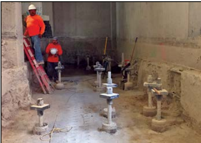
Project: Catalina Island Contractor: Condon-Johnson & Associates Location: Catalina Island, CA
