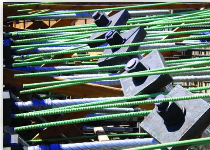
Project: Galena Creek Bridge Contractor: CC Meyers Location: Reno, NV
