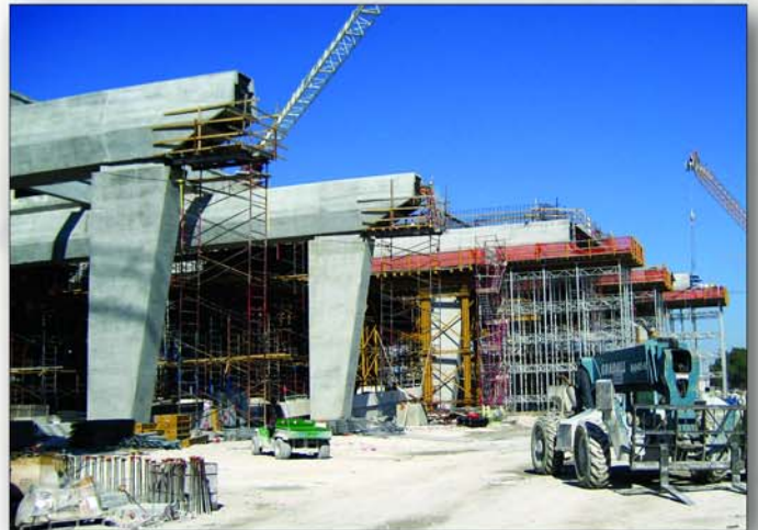
Project: MIC-MIA Connector Station Contractor: Turner Construction / VSL Location: Miami, FL
