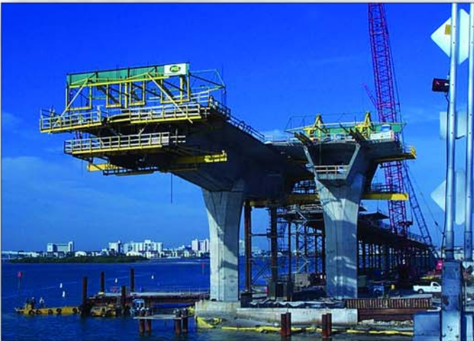
Project: Memorial Causeway Bridge Contractor: PCL / VSL Location: Clearwater, FL
