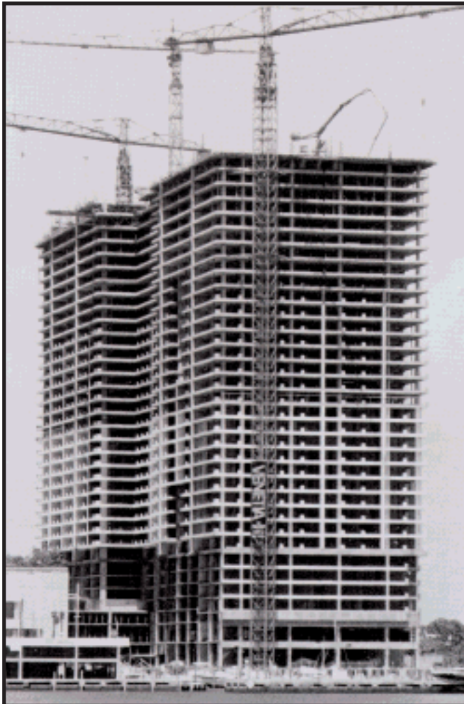
Plaza Ventia Condominiums - Miami, FL Sub-Contractor: Arrow Forming
